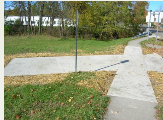
FY2008 – Village of North Lewisburg – Sycamore Street ADA Sidewalks
