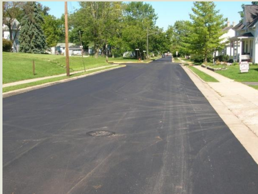
FY2008 – Village of Mechanicsburg – East Race Street Improvements
