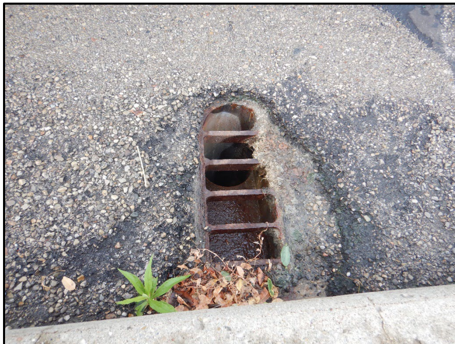
Photo 10 – Looking south at typical deck scupper detail. Note: multiple asphalt overlays.
