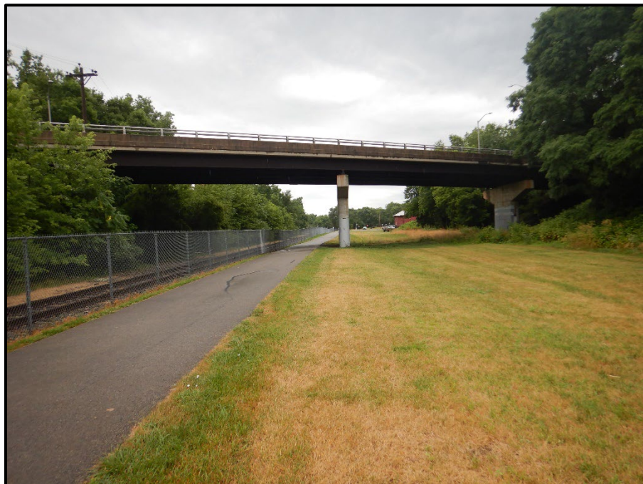
Photo 2 – Elevation looking north.
