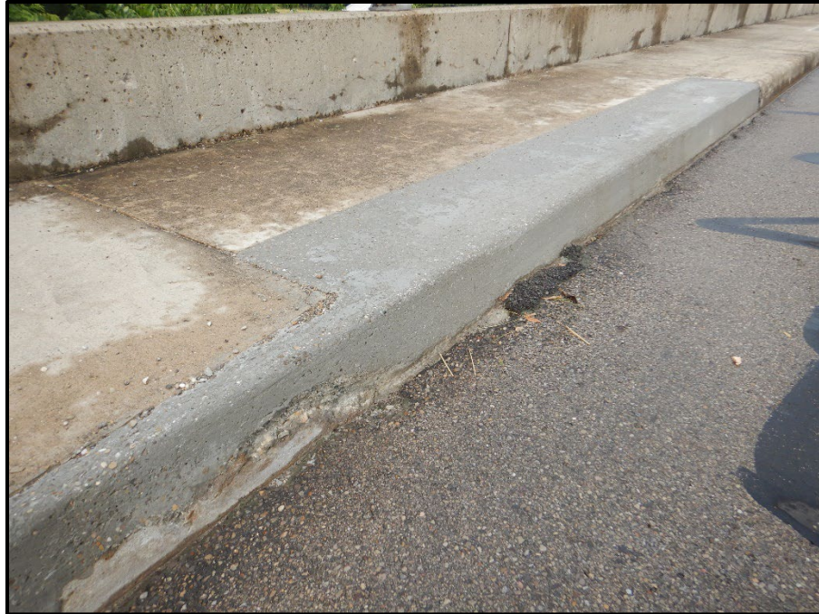
Photo 7 – Looking south at the sidewalk repair in span 3.
