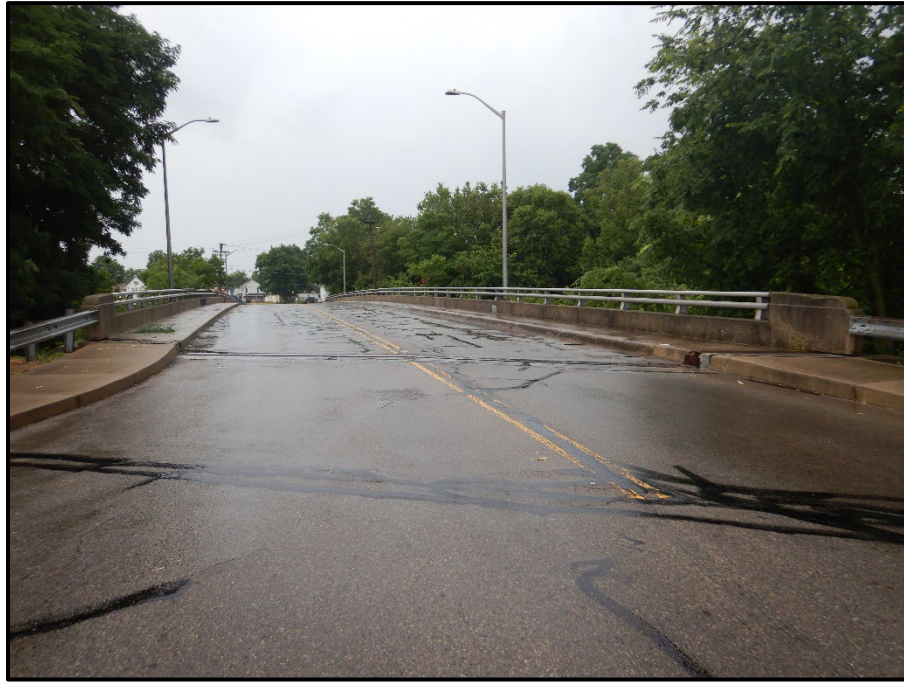
Photo 1 – End view looking east.
