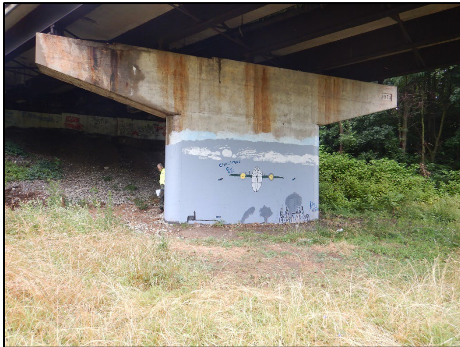
Photo 30 – Looking west at the elevation view of the Rear Pier.
