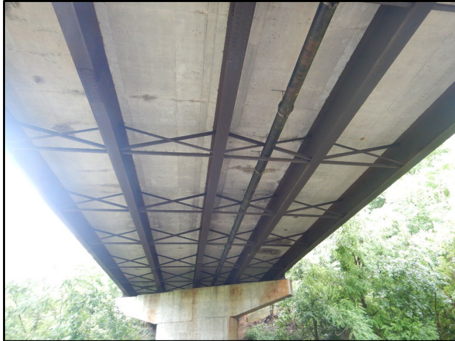
Photo 3 – Looking east at the typical underside of span 3.
