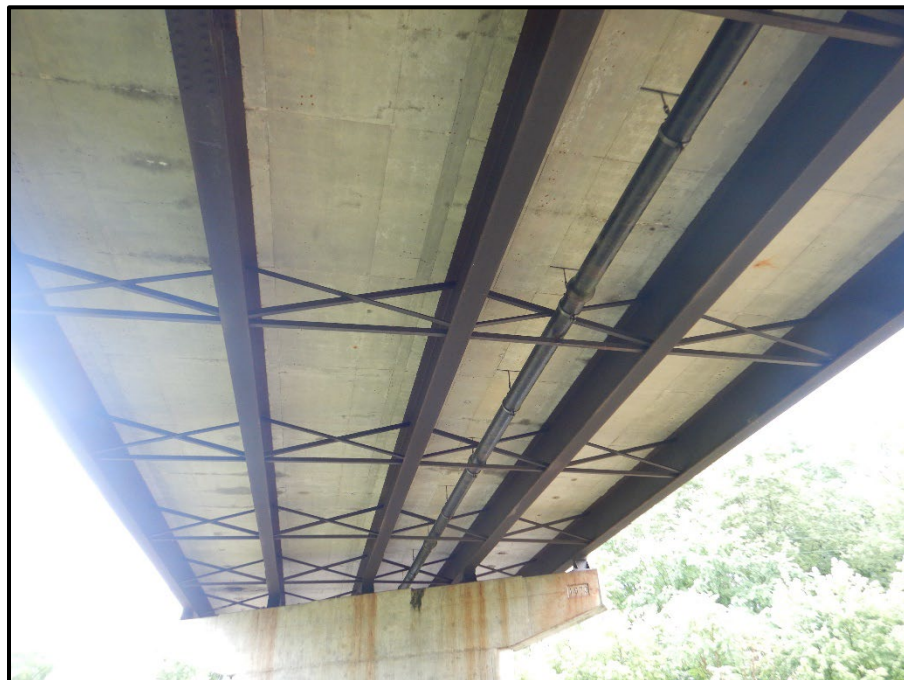
Photo 14 – Looking east at the underside of span 2.
