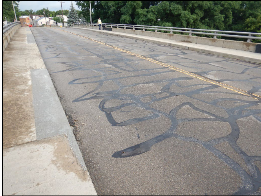
Photo 5 – Looking northwest at the typical wearing surface in span 3.
