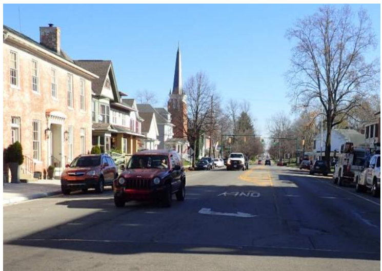
Photo 1: Faded Channelizing Line at Locust St
