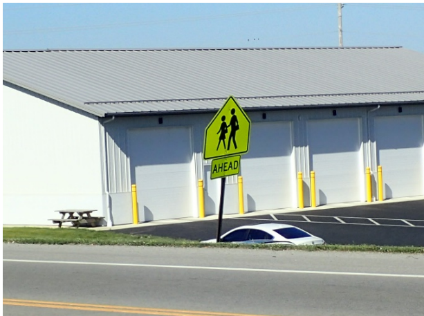
Photo 3: Improperly Mounted Sign
