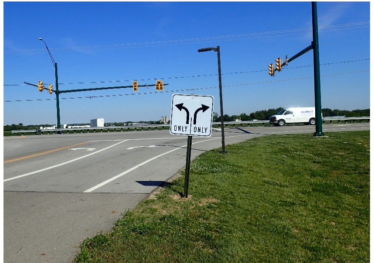
Photo 1: Improperly Mounted Lane Use Sign
