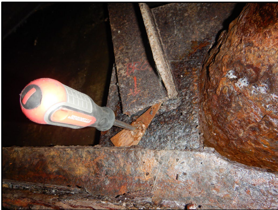
Photo 20 – Looking east at the end cross-frame between beams C and D at the Forward Abutment. Note: broken diagonal angle weld.
