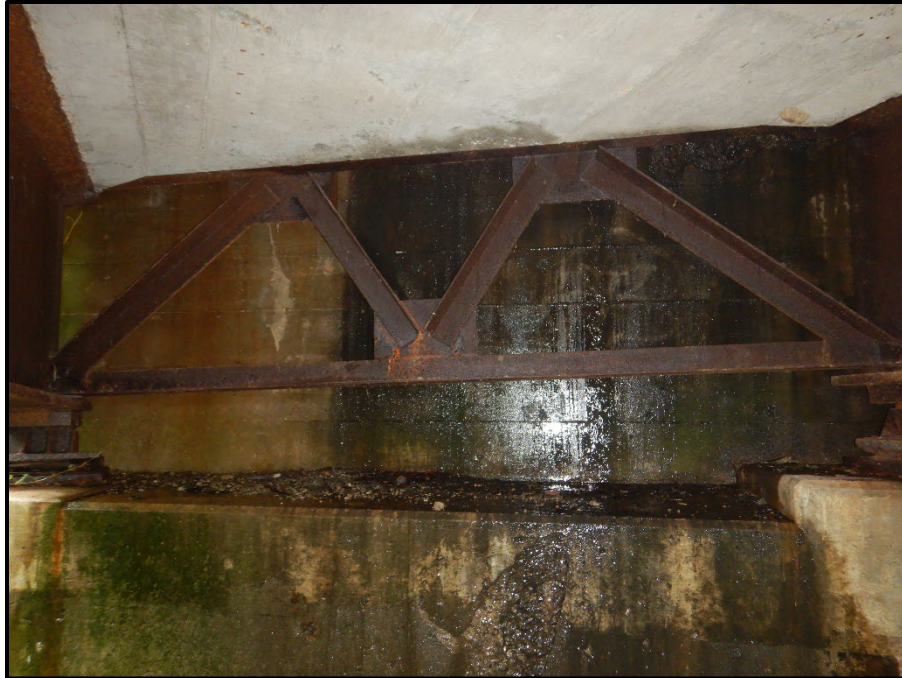
Photo 13 – Looking east at the end cross-frame between beams A and B at the Forward Abutment. Note: heavy surface corrosion exists on the end cross-frames due to water infiltration through the deck joint.
