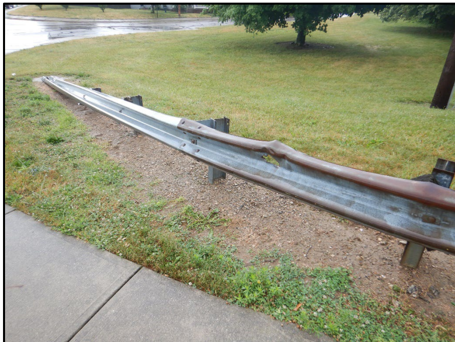
Photo 36 – Looking northwest at the northwest approach guardrail. Note: turn down end treatment.
