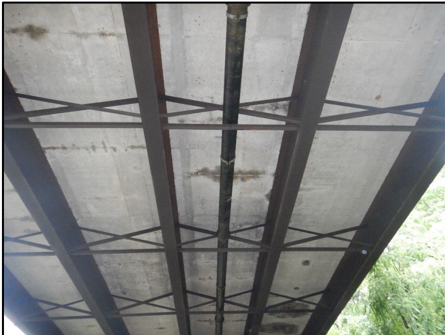
Photo 26 – Looking east at the water pipe running between beams C and D.
