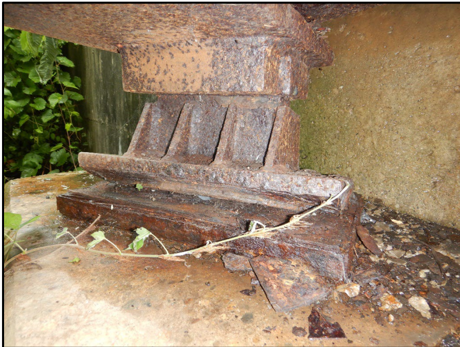
Photo 24 – Looking north at the rocker bearing under beam A at the Forward Abutment. Note: laminar corrosion exists to the masonry plate due to a leaking expansion joint.
