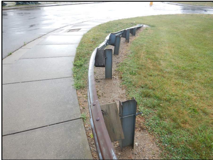
Photo 37 – Looking west at the northwest approach guardrail. Note: 5-foot-long section of impact damaged guardrail and multiple twisted and loose timber block outs.
