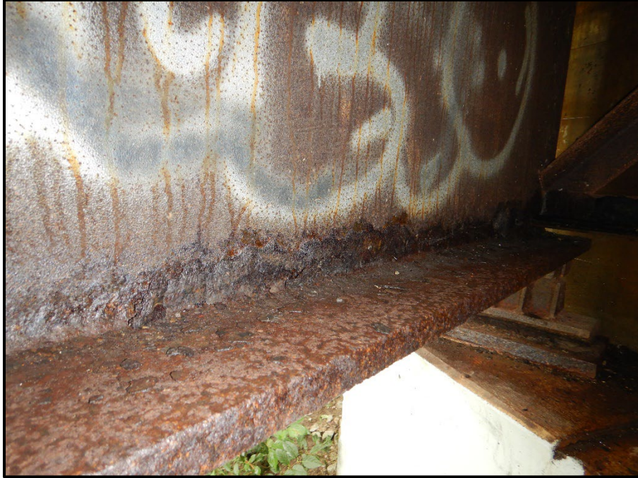
Photo 15 – Looking southwest at span 1 beam E at the Rear Abutment. Note: laminar corrosion typical on the end 4 feet the steel beams at both abutments.
