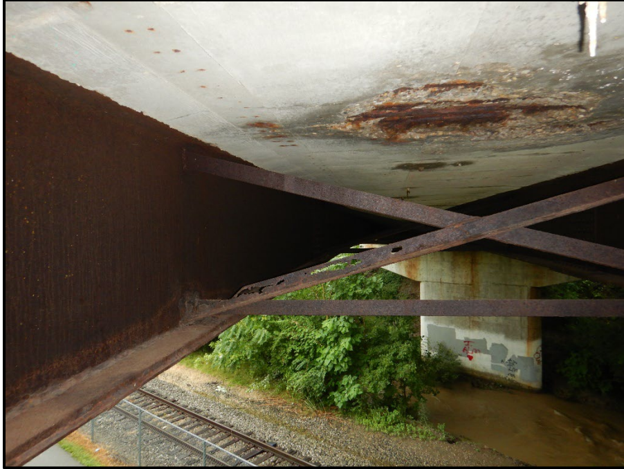
Photo 23 – Looking at span 3 intermediate cross-frame 10 between beams B and C near the Center Pier. Note: bottom of concrete deck spall and full depth corrosion holes exist in the cross-frame diagonal due to flow from the asphalt drain.
