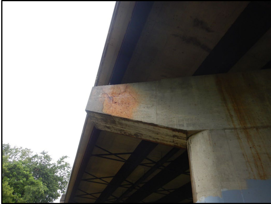
Photo 31 – Looking west at the south end, east face of the Center Pier cap. Note: multiple shear cracks emanating from the beam E bearing.
