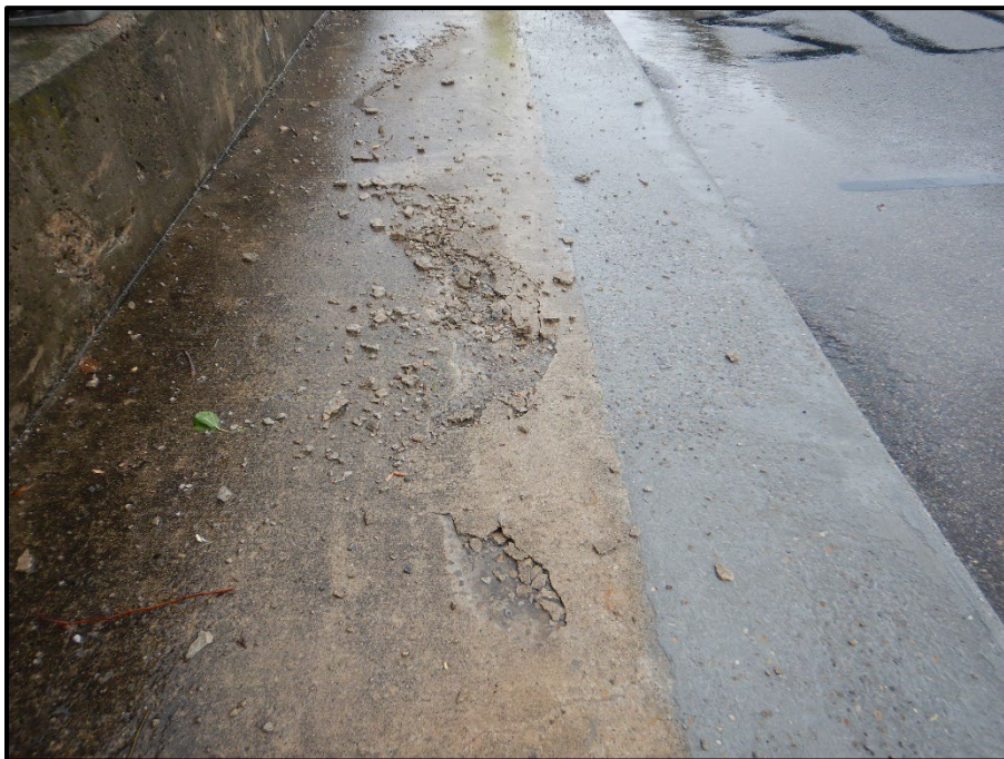
Photo 8 – Looking west at the south sidewalk in span 3. Note: 7-foot-long section of the sidewalk is scaling.
