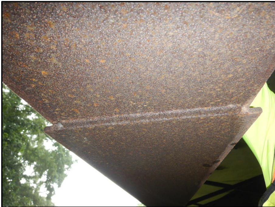
Photo 16 – Looking east at the moment plate on the bottom flange of beam A in span 1.
