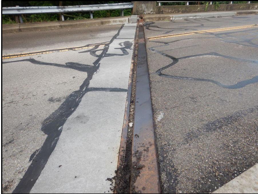
Photo 11 – Looking south at the sliding plate joint over the Rear Abutment. Note: soil and debris are accumulating in the joint.
