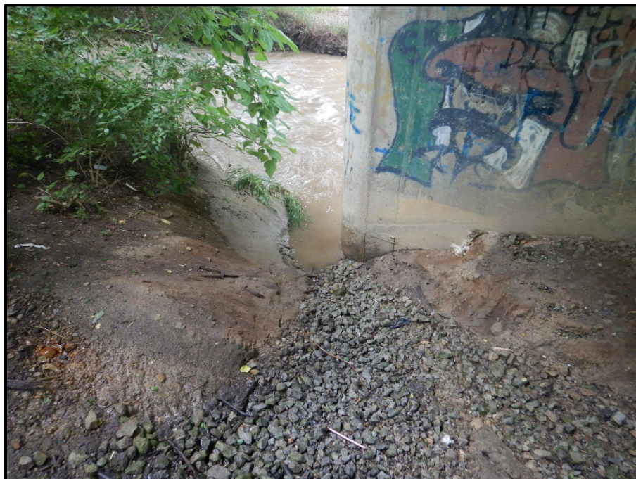
Photo 34 – Looking west at the scour hole at the end of an erosion ditch at the south end of the Forward Pier.
