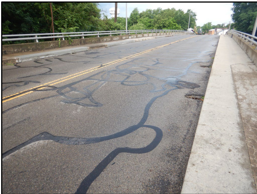
Photo 6 – Looking southwest at the typical wearing surface condition in span 1. Note: sealed map cracking throughout. Multiple locations of concrete sidewalk repair throughout all spans.
