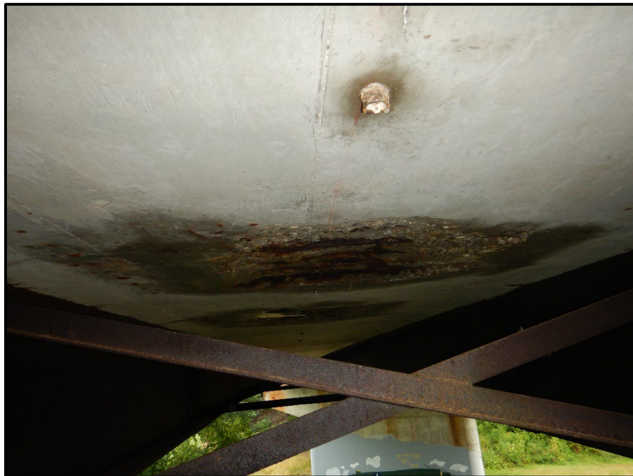
Photo 4 – Looking west at the underside of the deck in span 3 bay 4 near the Center Pier. Note: two 5-foot x 5-foot spalls with exposed reinforcing steel in the underside of the deck.
