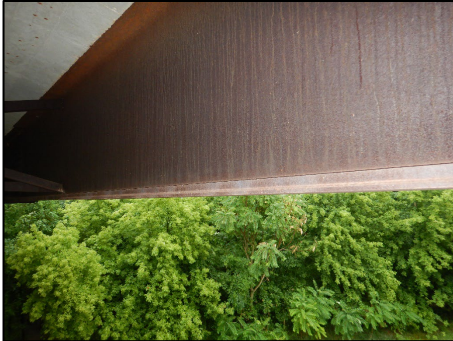
Photo 17 – Looking southeast at beam E in span 3. Note: moment plates are wider than the bottom flange.
