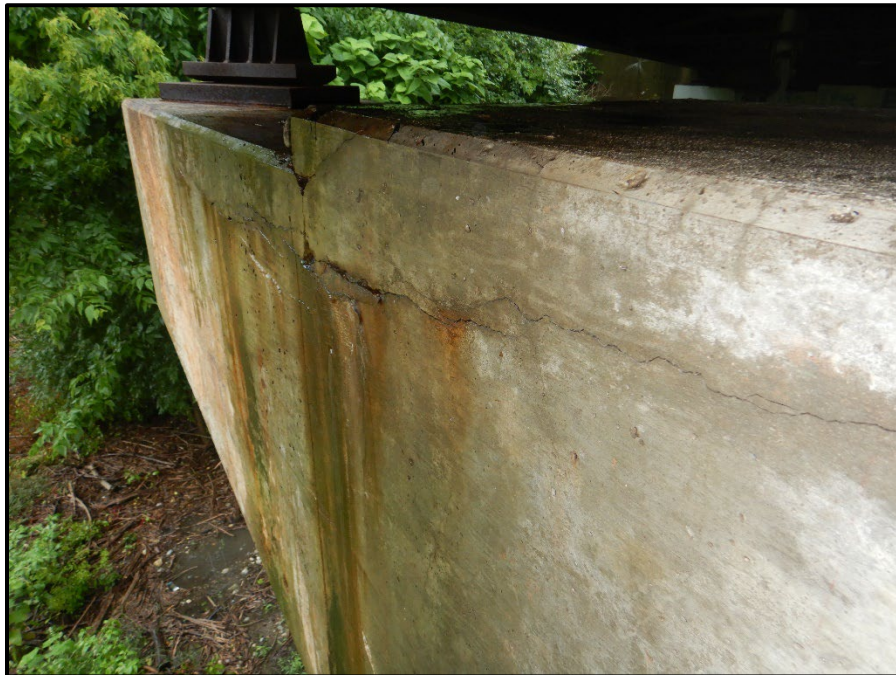
Photo 32 – Looking south at the south end, east face top corner of the Rear Pier between beams D and E. Note: 2-foot-wide x 4-foot-long x 16-inch-tall delamination caused by asphalt drain located directly above the cap.
