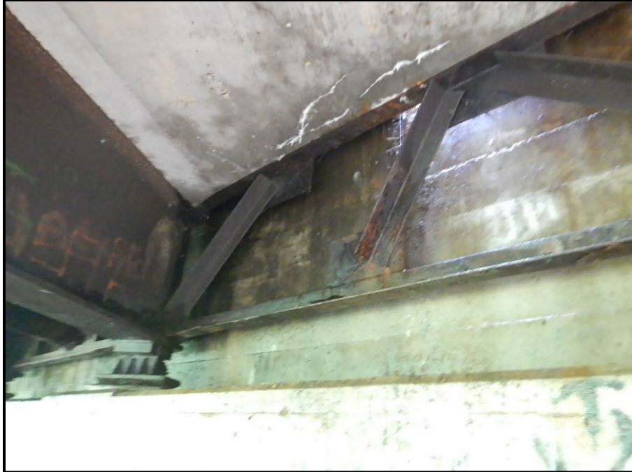
Photo 19 – Looking east at the end cross-frame between beams D and E at the Forward Abutment. Note: missing diagonal angle.
