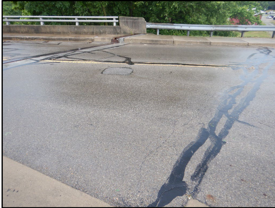
Photo 35 – Looking south at the west approach roadway. Note: multiple sealed transverse and longitudinal cracks in the approach roadway.
