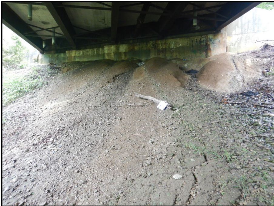
Photo 28 – Looking east at multiple erosion ditches formed by scupper drainage in embankment in front of the Forward Abutment. Similar conditions are present at the Rear Abutment embankment.
