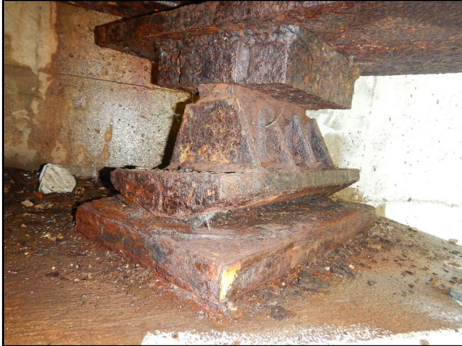
Photo 25 – Looking northwest at the beam A rocker bearing at the Rear Abutment. Note: laminar corrosion with up to 1/8 inch loss to the masonry plate and bearing interface.
