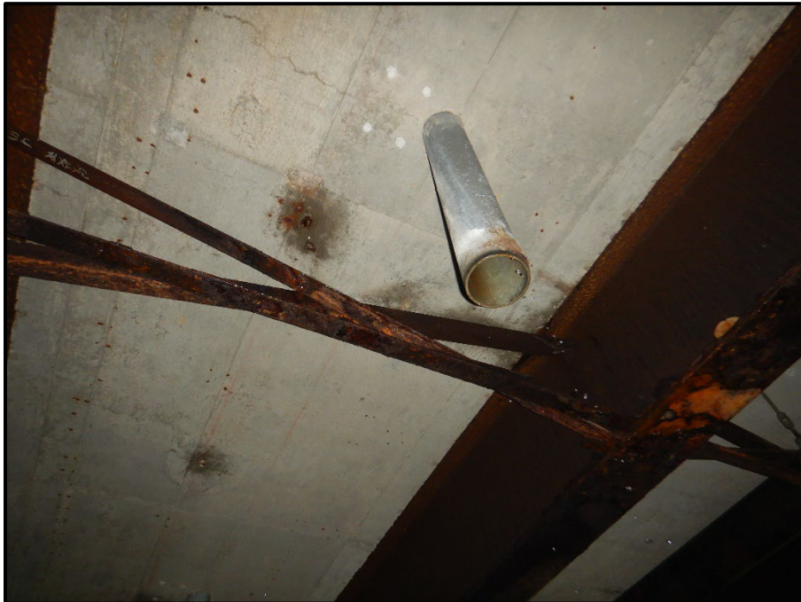
Photo 22 – Looking west at the scupper drain and asphalt drain in span 4 between beams D and E at cross-frame 17. Note: asphalt drain is directly over intermediate cross-frame and drainage flows onto diagonal member and down to the bottom flange of the beam.
