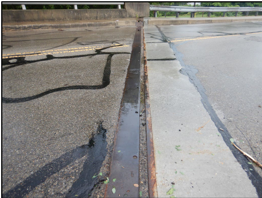
Photo 12 – Looking south at the sliding plate joint over the Forward Abutment. Note: soil and debris are accumulating in the joint.
