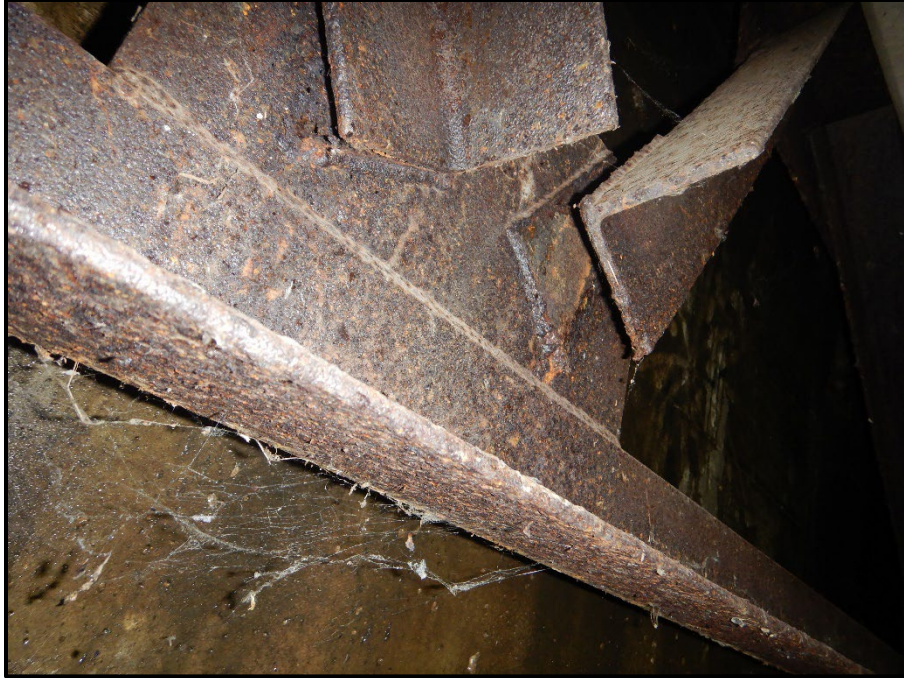
Photo 21 – Looking east at the end cross-frame between beams B and C at the Forward Abutment. Note: broken diagonal angle weld.
