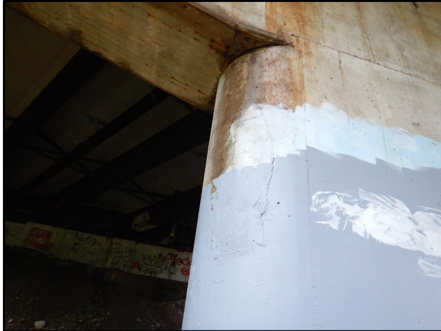
Photo 33 – Looking west at the south end of the Rear Pier wall. Note: 4-foot-tall x 2-foot-wide delamination caused by an asphalt drain discharging onto the top of the pier cap.
