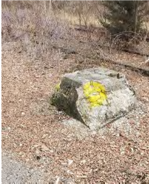
Photo 3: Concrete Light Pole Foundation
