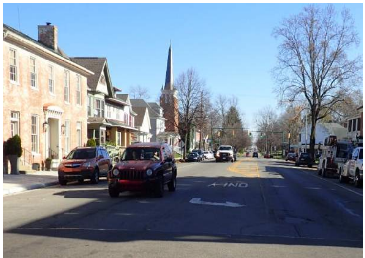
Photo 1: Faded Channelizing Line at Locust St
