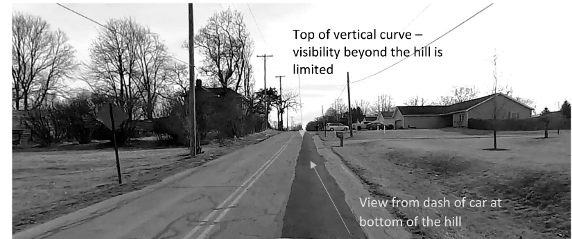
Exhibit 3.4 – Childrens Home Road heading east looking towards vertical curvature limiting sight distance
